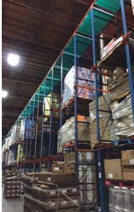
*Thermal Energy Storage modules installed on top crossmember of the racking structure. (Photo courtesy of Viking Cold.)*
